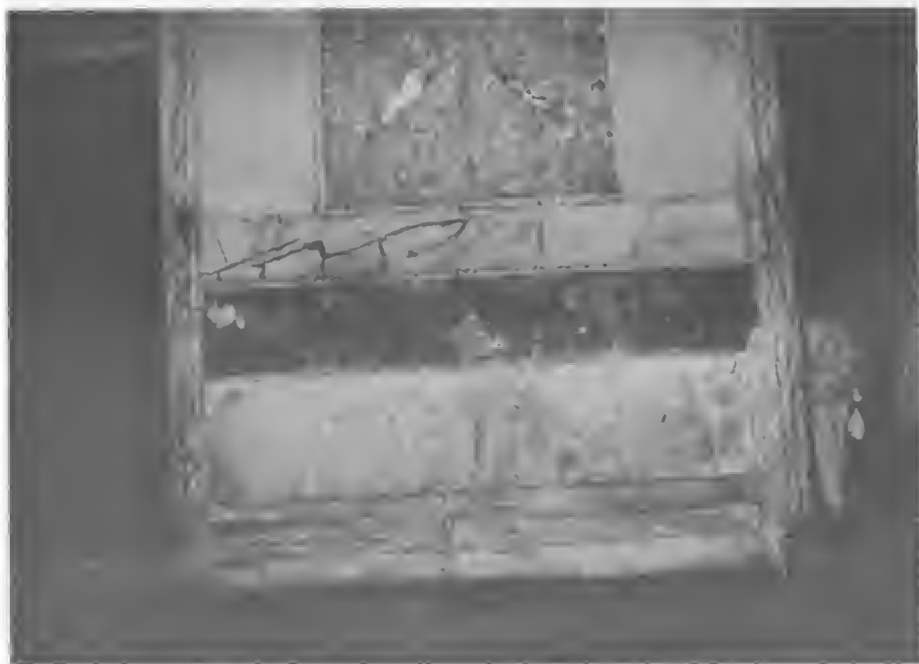
FIG. 7. — View of the wall with cross no. 9 on plan at ground level.
